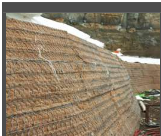
TERRAMESH SYSTÉM - DETAIL
